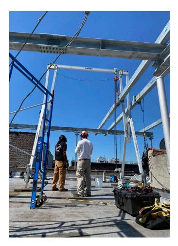
The solar panels are installed onto older infrastructures, meaning that Urban Energy were conscious of using large, heavy lifting equipment onto the roofs and therefore required a lightweight system, like the ones that REID Lifting Inc could offer.
